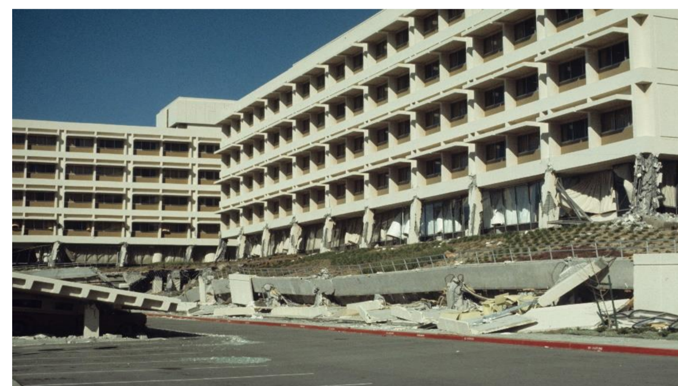
Fig. 1 – Soft Storey Collapse of Olive View Hospital 1971 San Fernando earthquake .
