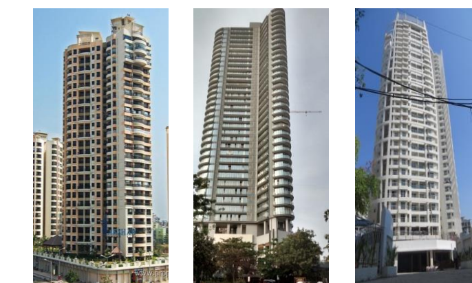
Figure: Examples of typical high-rise buildings
