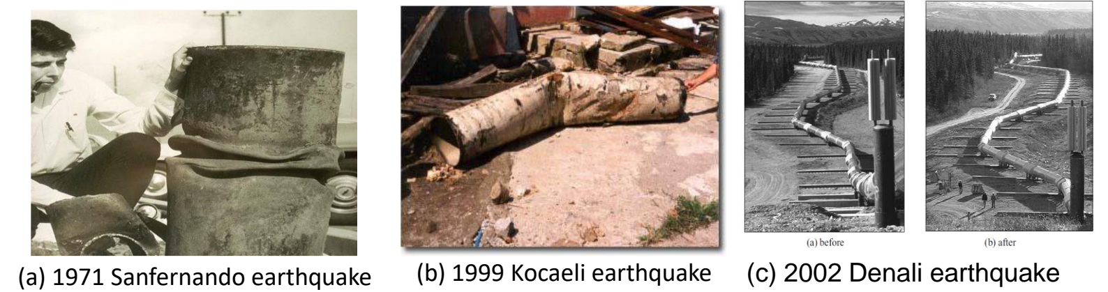
Fig 1. Failure of pipelines during past earthquake
